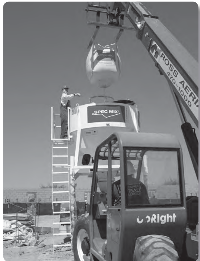
Solution: Loading a silo system
