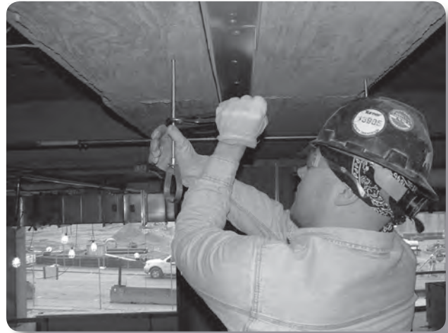
Problem: Tightening conventional nut on all-thread
