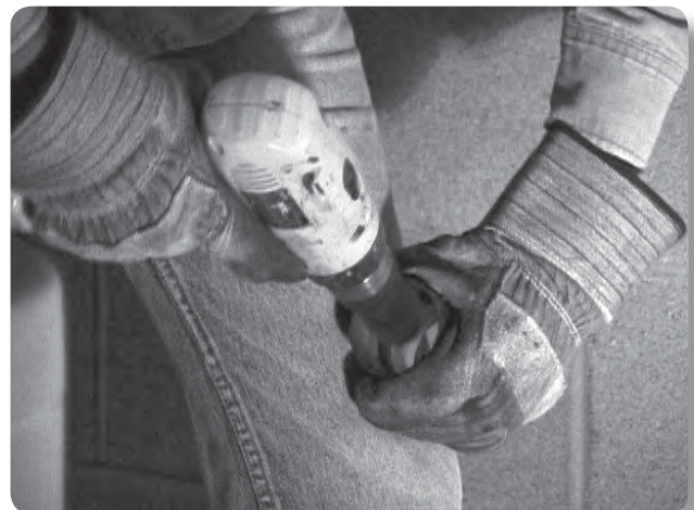
Solution: Using wire brush with power driver
