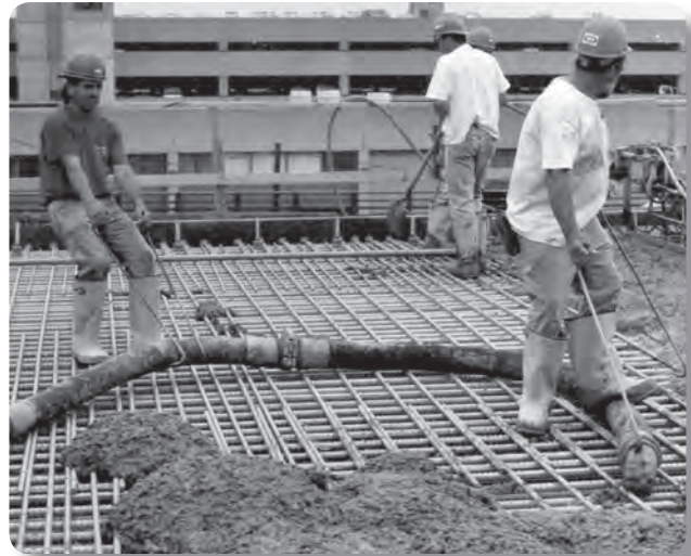
Problem: Pulling concrete hose without skid plate
