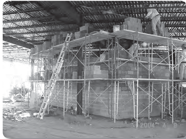
Problem: Conventional unguarded frame scaffolding
