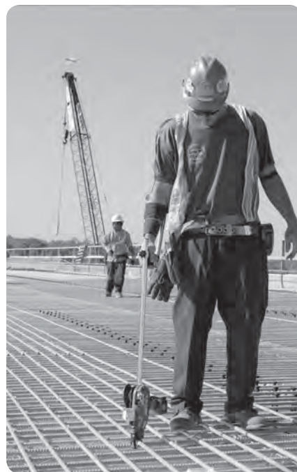
Solution: Rebar-tying tool with extension handle
