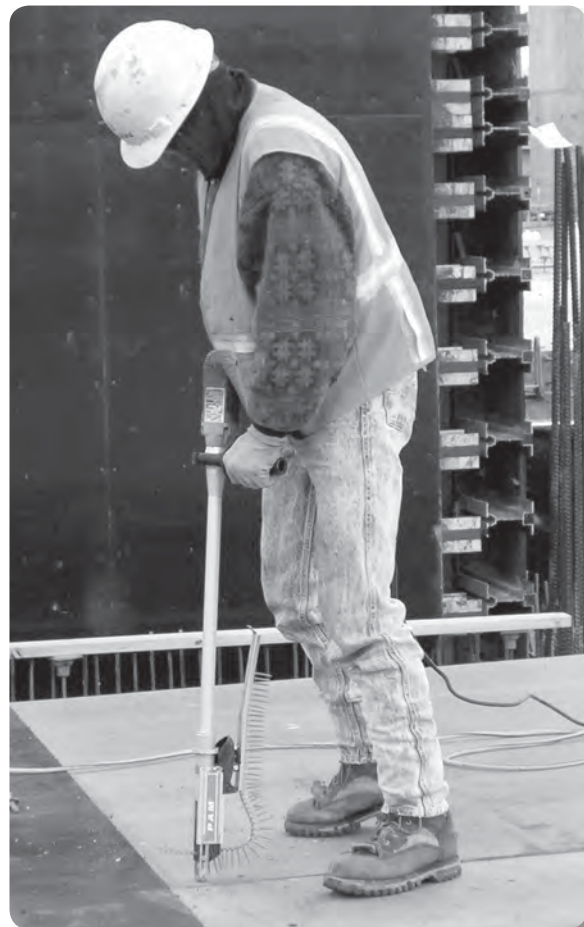
Solution: Autofeed stand-up screw gun
