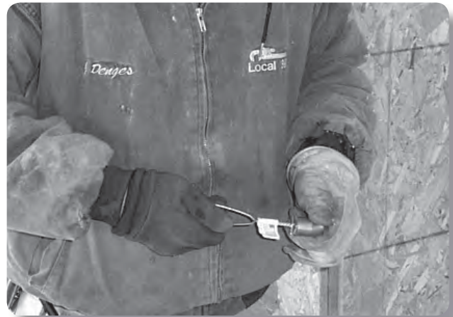
Problem: Brushing copper tube by hand
