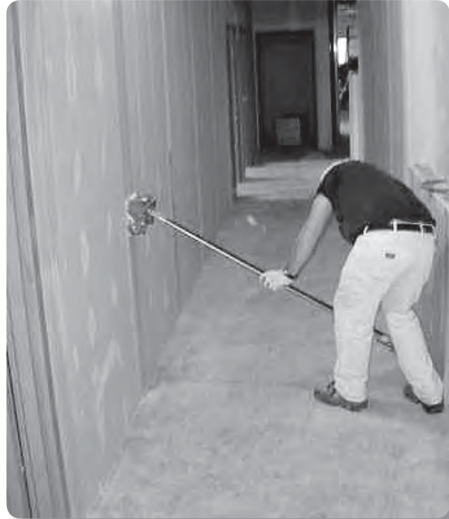
Problem: Hand drywall finishing with mudbox
