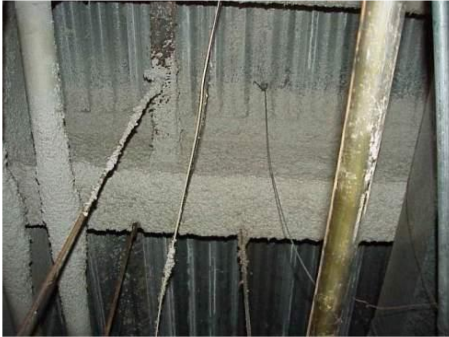
Sprayed-on fireproofing material
