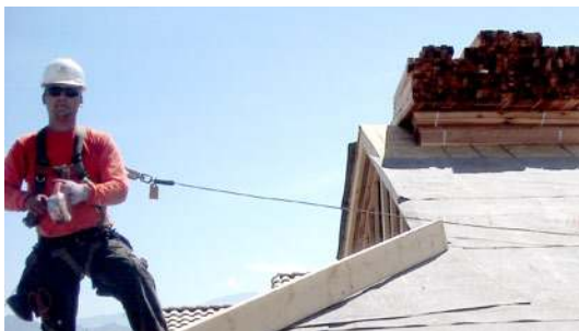
Photo courtesy of ACTA Safety & Peterson Dean Roofing
